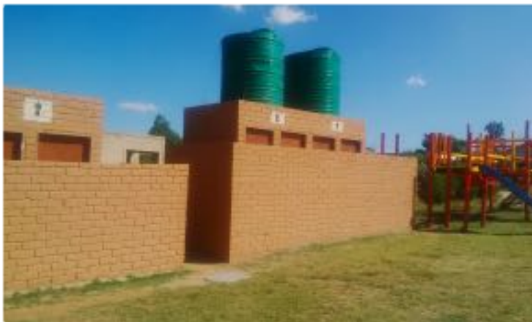
MAC Water system (we also have our own filtration, disinfection system and booster pump controller )
